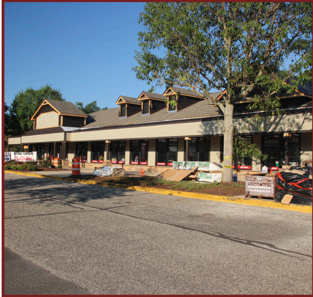
Remodeling being done in the Village of Taunton Forge
