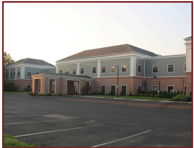
Medical Building at 103 Old Marlton Pike (After Remodel)
